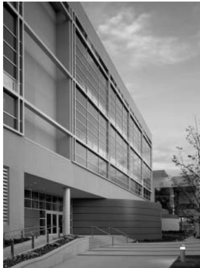
Figure 3. The perimeter windows contain low-E glazing, as do the special skylights.
