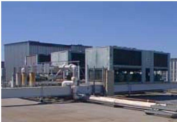
Facility B.2 48°F Chilled Water System
