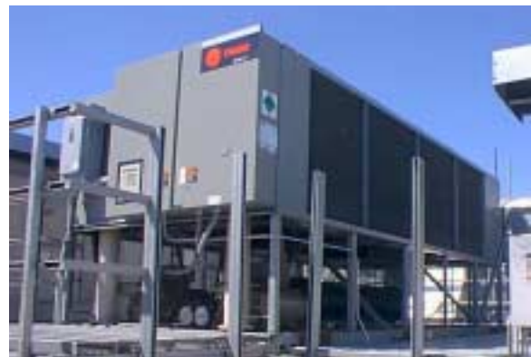
Facility B.2 40°F Chilled Water System
